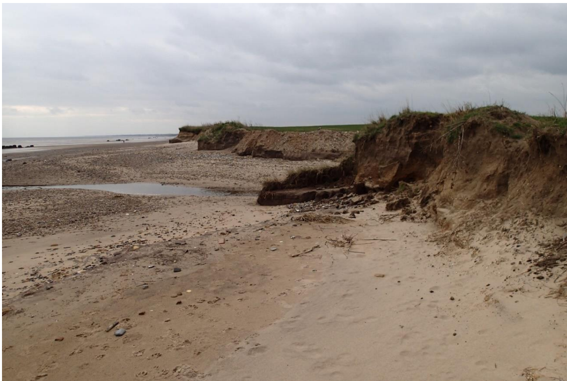
Plate 7. Fresh water run off. T3 upper-shore (site ref 277)
